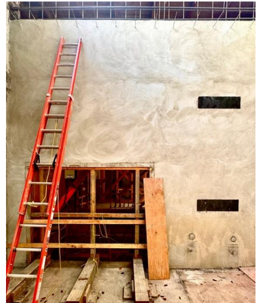
Reinforced concrete shear walls for future study rooms at the University Branch.
