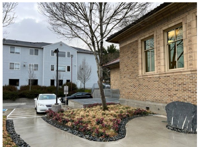
New ADA walkway at Douglass-Truth Branch
